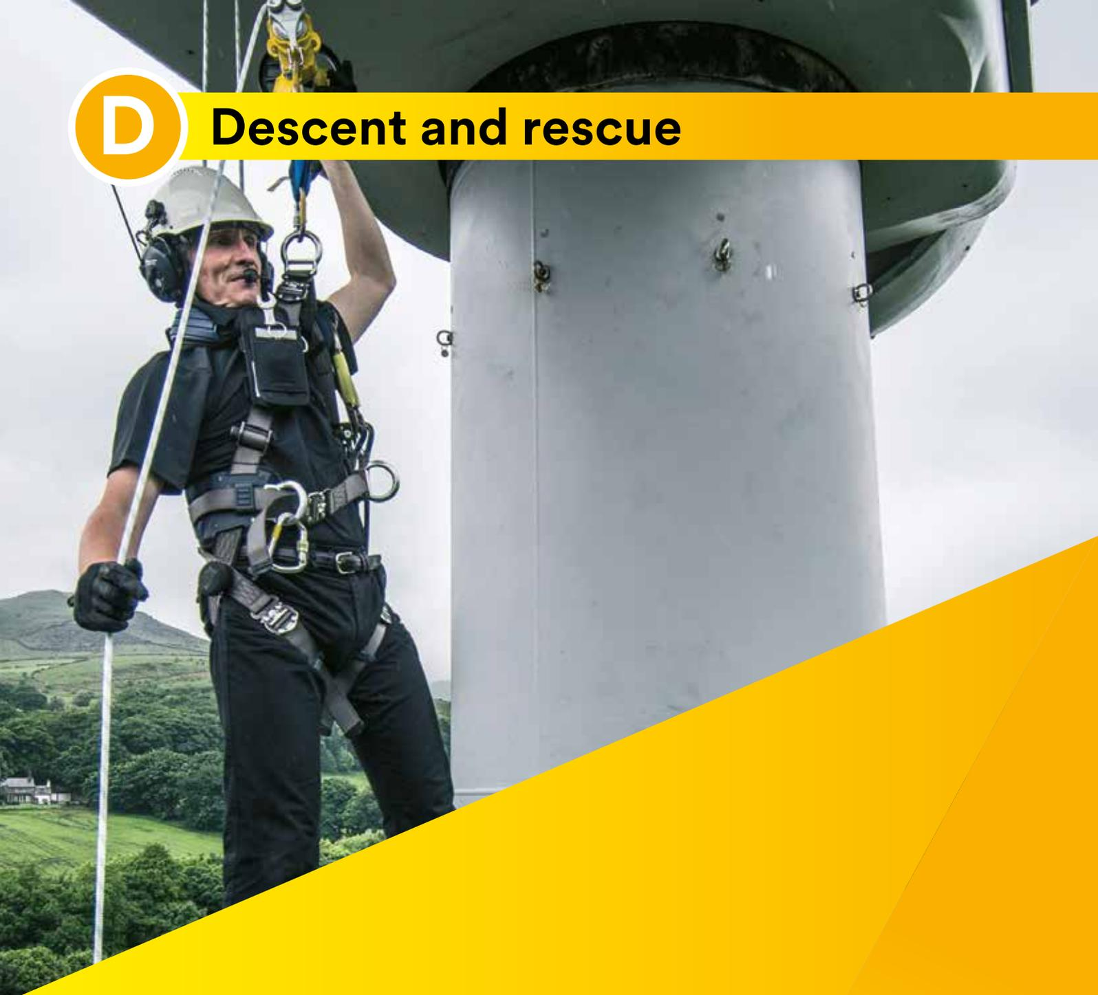
**Descent and rescue devices are used to raise or lower a fallen or injured worker to safety or retrieve him from a confined space.**
